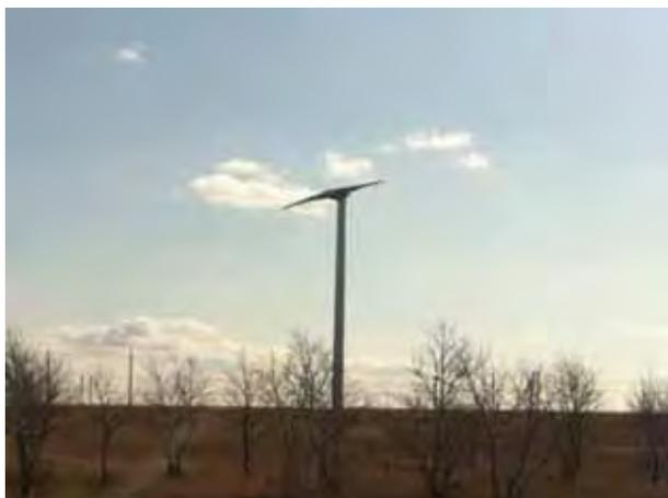
**Figure 3-3 | Two-blade WTG** (Ming Yang)
