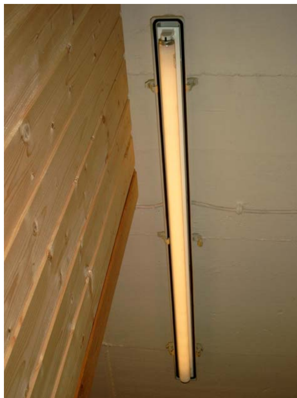
Fig. 3.16: Removal of the cover reveals: One of the two lamps is still of the old T12 type and still working well
