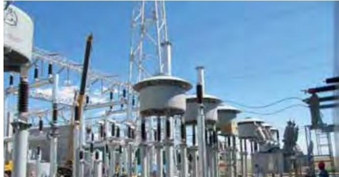
Figure 4-6 | 750 kV CSR at the Dunhuang substation, NW China (SGCC)
