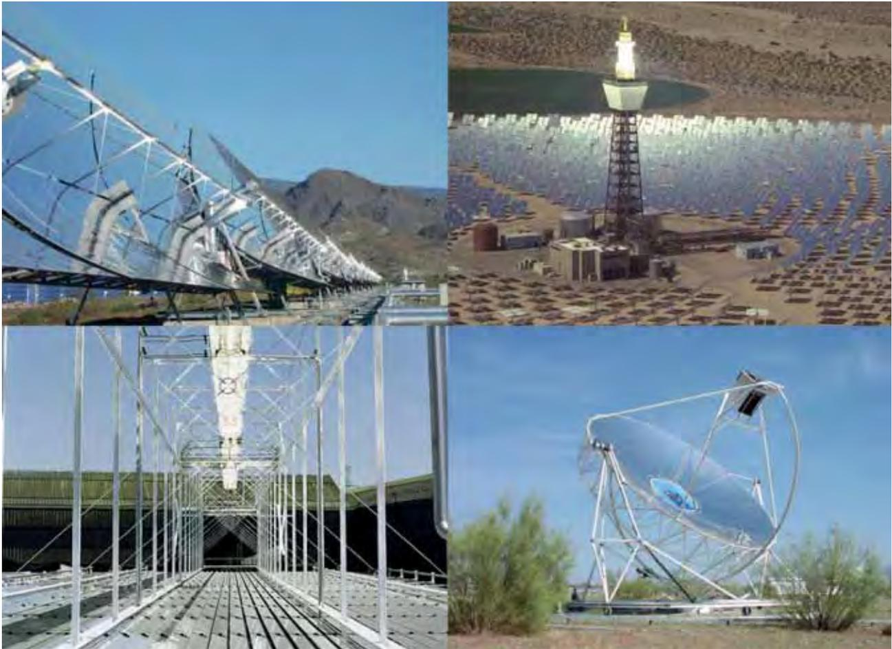
(a) Parabolic trough system
