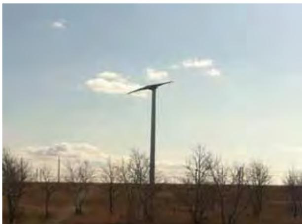
**Figure 3-3 | Two-blade WTG** (Ming Yang)
