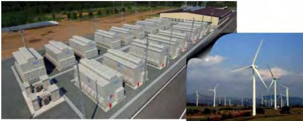
**Figure 5-7 | JWD’s wind and NAS battery hybrid system in Japan (NGK)**
