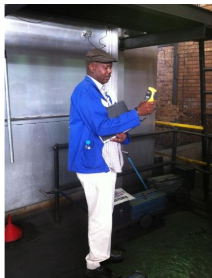
Figure 6 – Thermal imaging is non-intrusive and so safe and quick to use. (Atkins)
