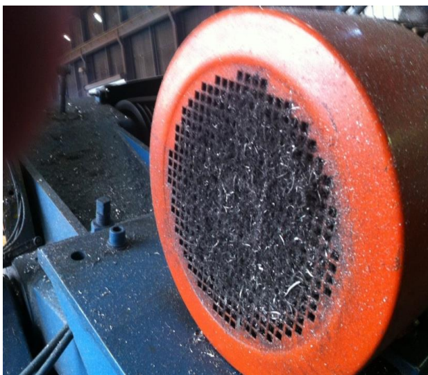
Figure 5 – Partially blocked fan on an induction motor in a metal processing plant. (Atkins)
