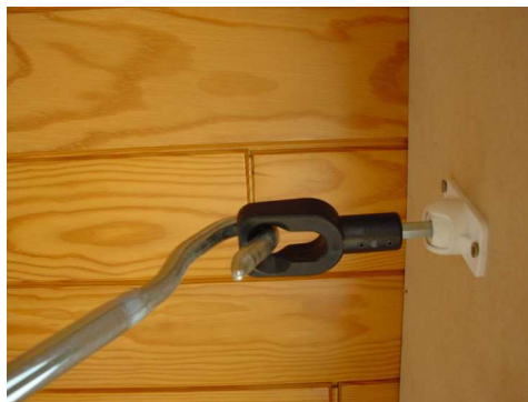
Figure 3: A mechanical emergency handle for an automated roll-down shutter might not be pretty, but the safety of the occupants takes precedence. (Illustration source: E&D Systems)
