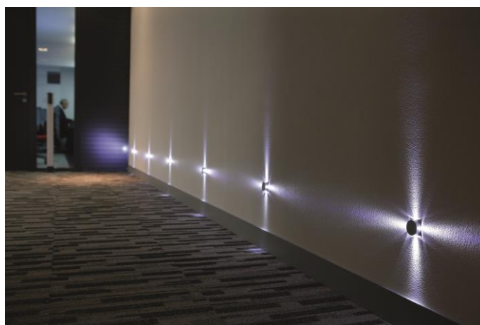
Figure 3: This indirect orientation lighting avoids glare. (Illustration source: Deltalight)
