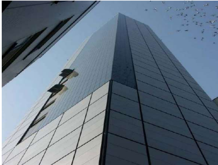
Figure 3 Example of PV integrated in facade of an office building(Würth Solar) [1]
