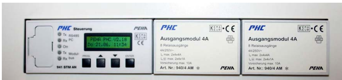
Figure 13: One input module and three output modules (3 x 8 x 4A) are used in the service flats. (Illustration source: Peha Belgium)
