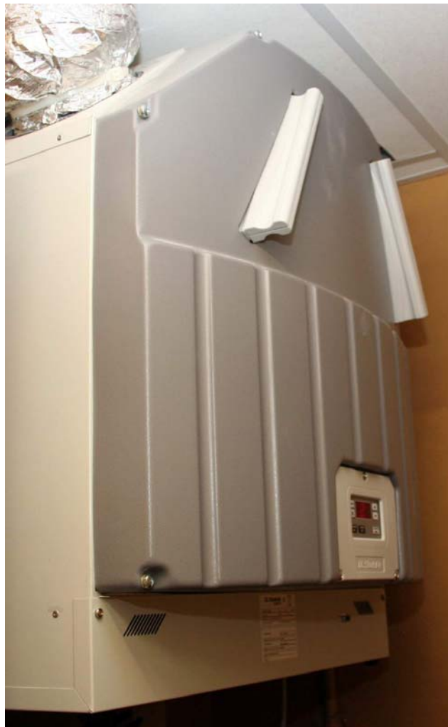
Figure 3: The ventilation unit with heat recovery (Illustration source: E&D Systems)
