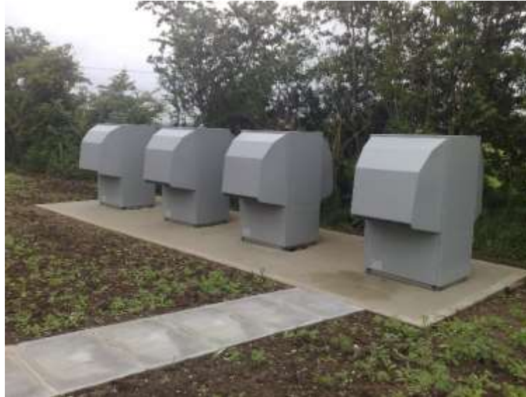
Figure 5 – 4 x 60kW Dimplex Air Source Heat Pumps providing heating, cooling and domestic hot water to an old people's home in the UK (reproduced with the permission of Nic Wincott).
