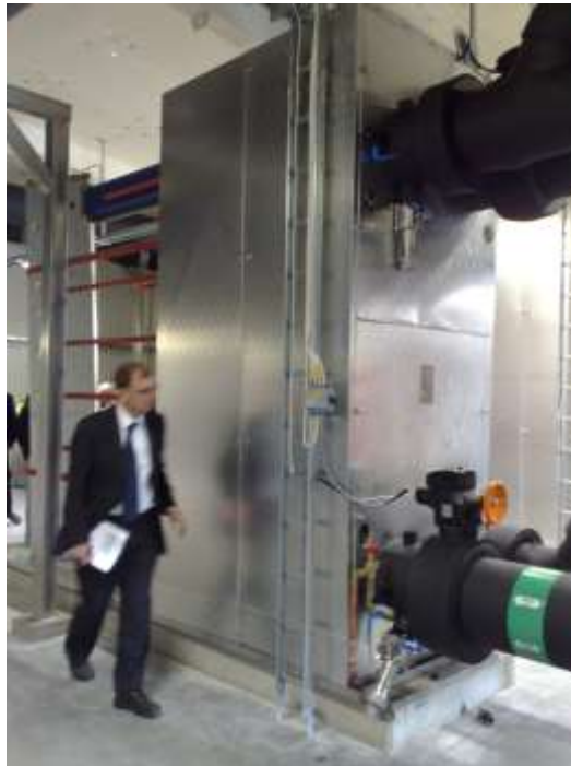
Figure 13 – Large Heat Exchanger used to deice the aircraft stands and to pre-heat or pre-cool incoming air to the terminal buildings at Arlanda Airport Stockholm ((reproduced with the permission of Nic Wincott).
