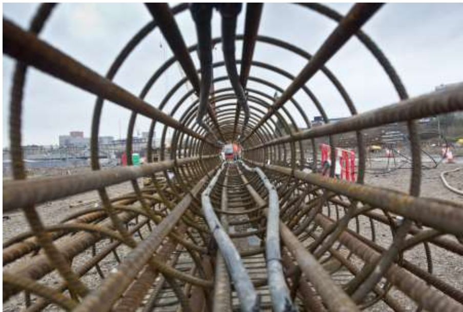
Figure 3 –Thermal Pile cage ready for installation (reproduced with the permission of Nic Wincott).
