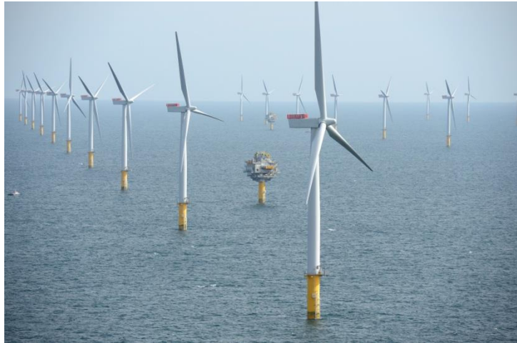
Figure 6—Offshore wind farm [8]
